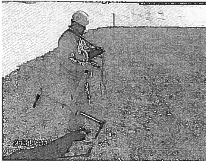
Leak location surveyor and equipment
