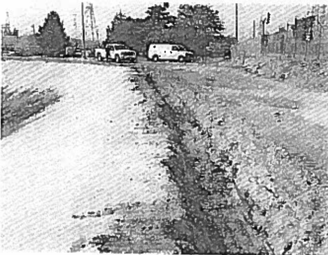
North anchor trench
