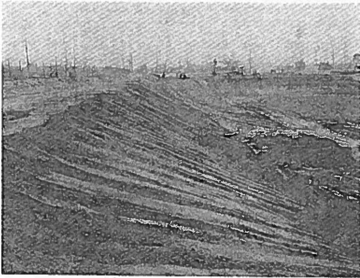
North side slope looking east
